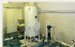
Auto water supply system of IIF Mitaka Card Center
