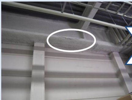
partial damage off fireproof
