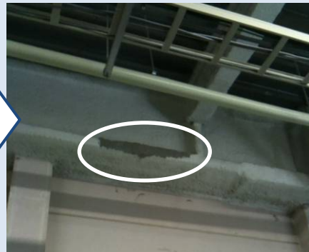
After repair of fireproof ( Using refractory fillers )
